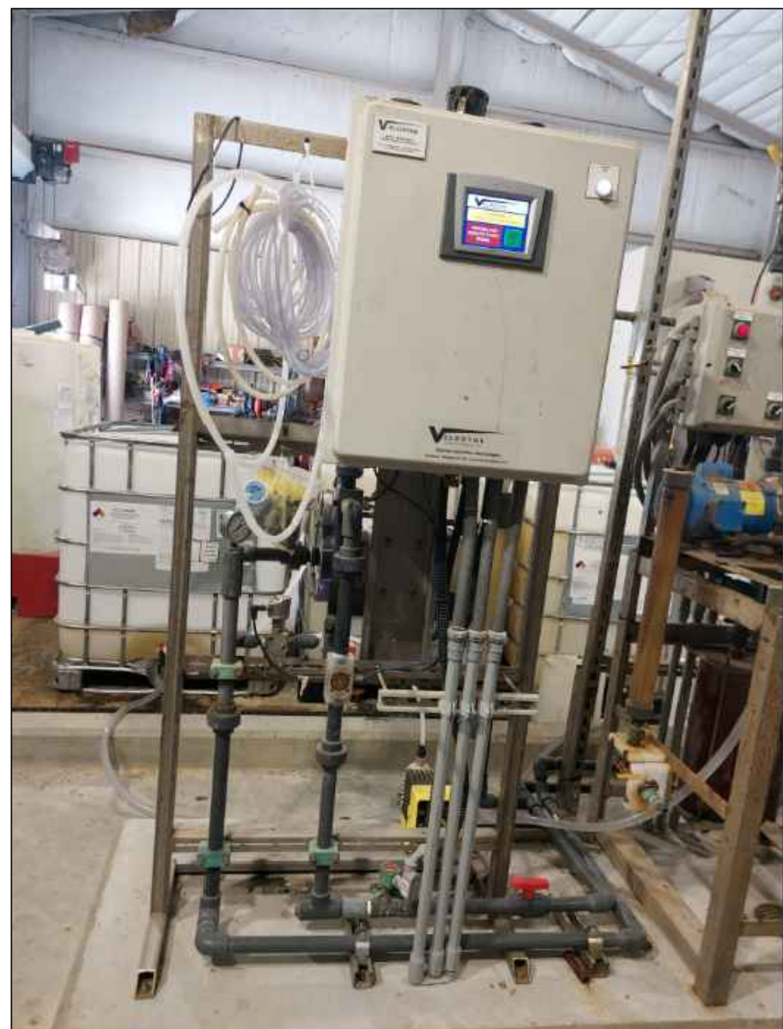
EXISTING POLYMER SKID - TO BE DEMOLISHED
