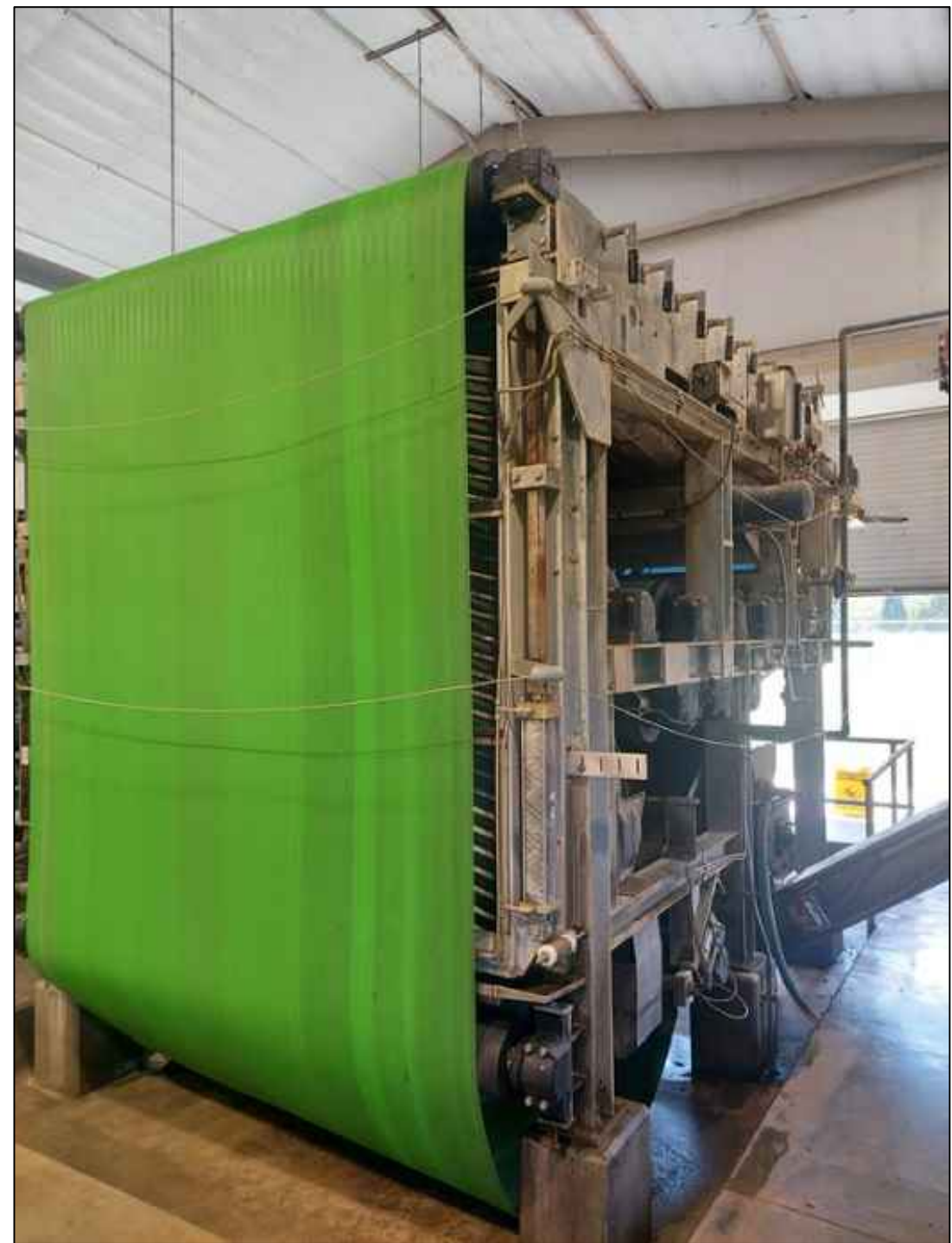
EXISTING BELT FILTER PRESS - TO BE DEMOLISHED
