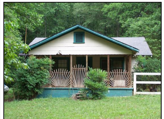
Inappropriate addition of a balustrade where none historically existed in an incompatible style.
