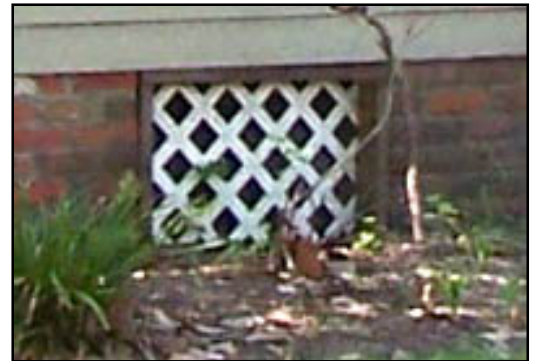
Appropriate use of lattice panel to screen foundation without covering brick piers.
