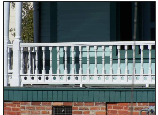
Turned and jigsawn woodwork on the porch.
