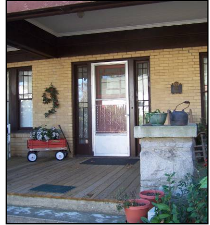
Inappropriate raw aluminum storm door.
