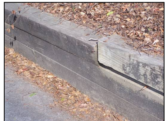
Wood is an inappropriate material for a retaining wall.
