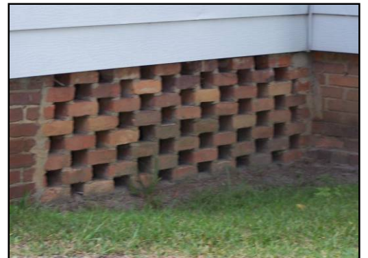
Appropriate maintenance of historic brick latticework infill.
