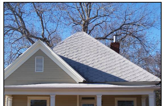
Historic roofing materials, such as these diamond-shaped asphalt shingles, should be retained, maintained, and replaced in-kind as needed.
