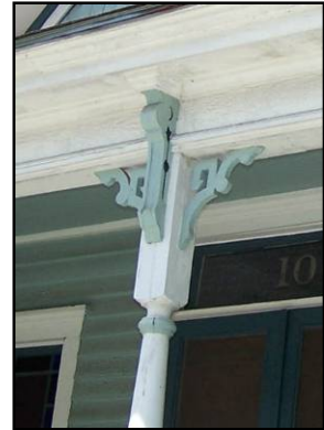
Appropriately maintained porch support with decorative bracket.
