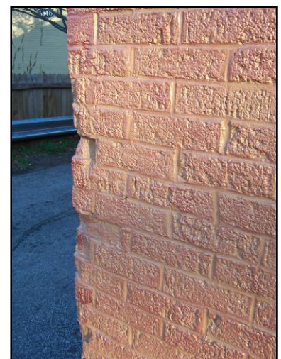
Inappropriately repointed masonry with incompatible mortar joints and mortar composition.
