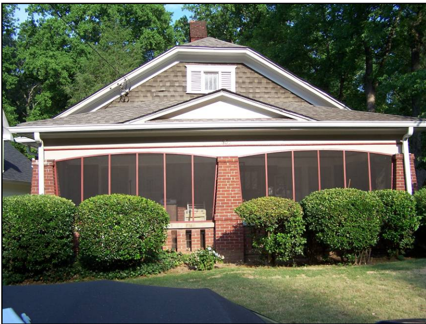
Appropriate enclosure of a porch with screening material in minimal wood framing.
