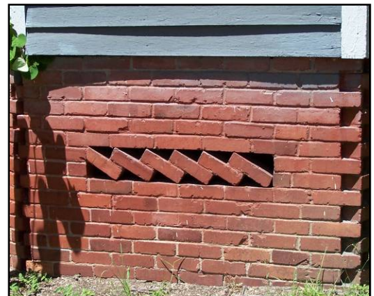
Appropriate maintenance of continuous brick foundation with decorative venting.
