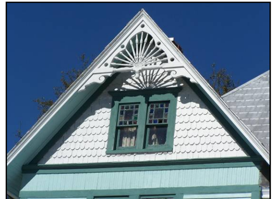
Complex spindlework, multi-light upper sash, and textured wall surfaces.
