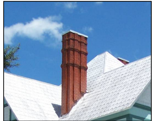
Maintain and repair historic chimneys and their decorative features, such as corbelled brickwork.
