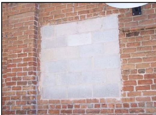
Damaged or deteriorated masonry should be replaced in-kind, rather than using another material.
