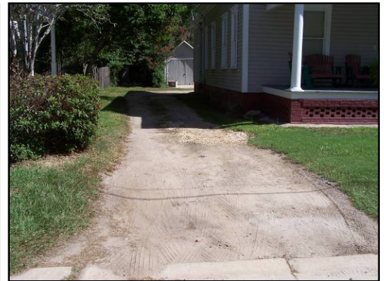
Appropriate driveway, located within the side yard, using permeable stone and sand surfacing.
