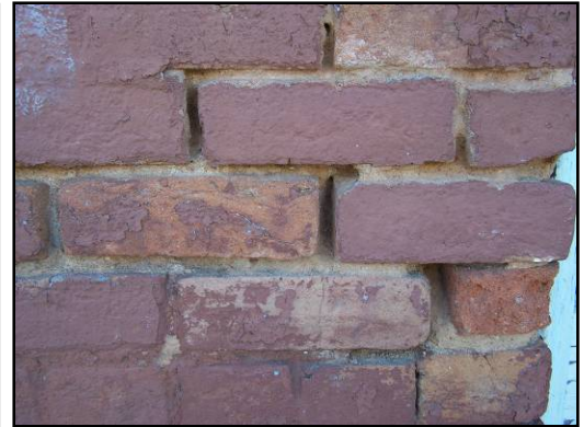
Crumbling mortar should be repointed.
