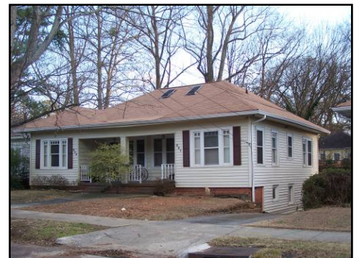
Inappropriate placement of a skylight on the front slope of the roof.
