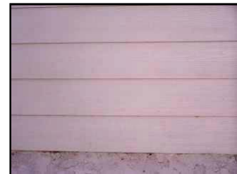
Fiber Cement Siding (Hardieboard) may be used for substantial rehabilitation projects of a significantly deteriorated building in Subarea II.
