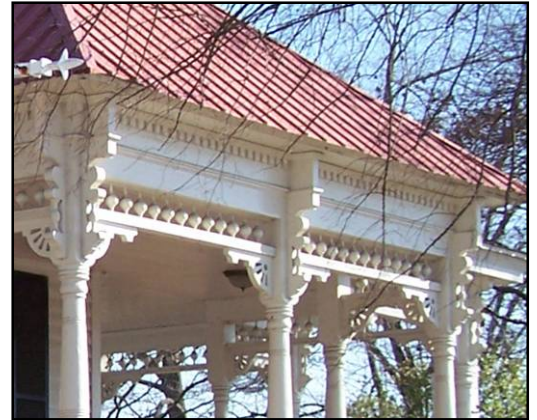
Standing-seam metal is an appropriate replacement material for asphalt shingle roofs for most houses within the historic district.
