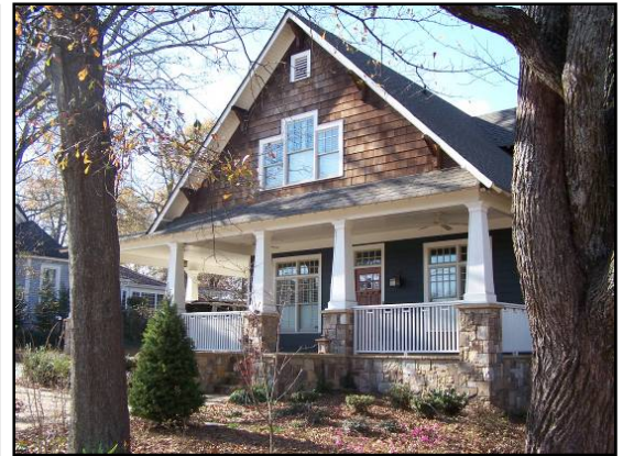
New construction using appropriate materials, including wood sash windows, fiber cement siding, and stone veneer.
