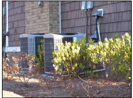
Condensing units and other mechanical equipment should be located on secondary elevations and screened with landscaping.
