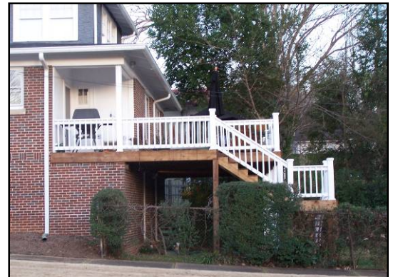
Appropriate placement of wood exterior stairs on the rear of a building.
