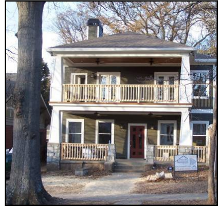
Inappropriate use of a wooden balustrade on a Craftsman-style porch.
