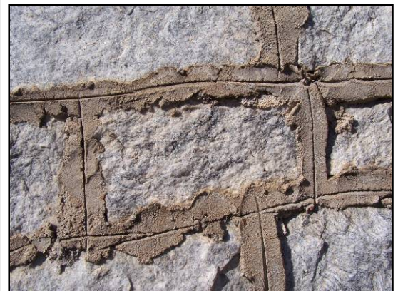
Inappropriately repointed masonry with incompatible mortar joints and mortar composition.
