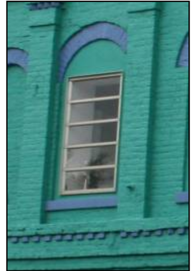
Inappropriate rectangular window in arched opening.
