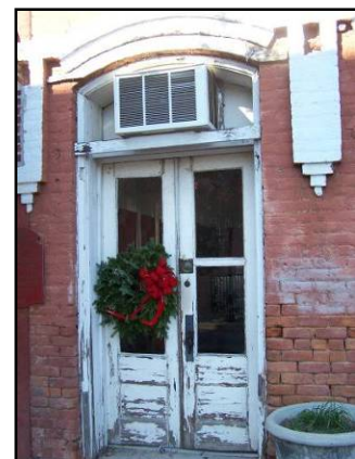
Inappropriate installation of an air-conditioning unit within a transom window.
