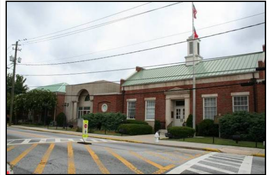
Standing-seam metal roofs are appropriate for historic buildings.
