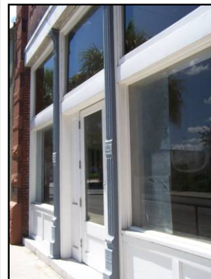
Inappropriate replacement of display windows with contemporary design.
