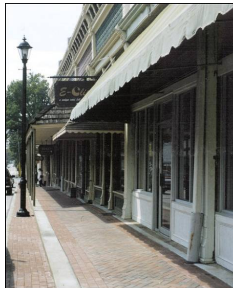
Inappropriate awning supported by sidewalk poles.
