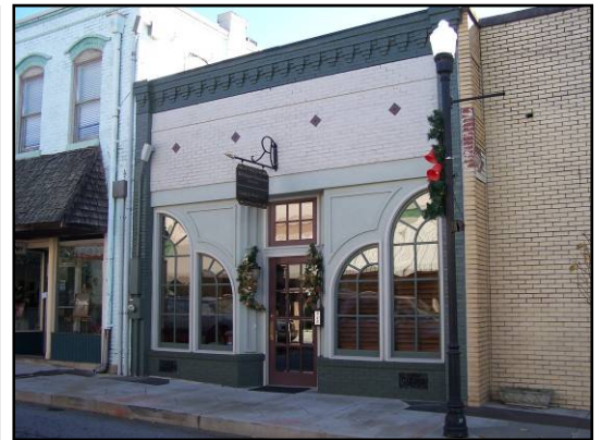
Inappropriate replacement of display windows with contemporary design.
