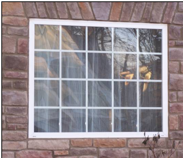
Flush or snap-in muntins are not an appropriate material for new construction.
