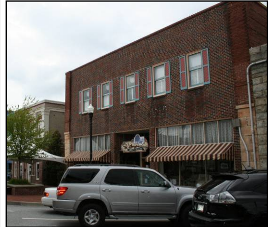
Inappropriate use of shutters.
