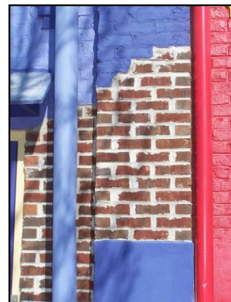
Replacement masonry units with compatible size, shape and chemical composition.
