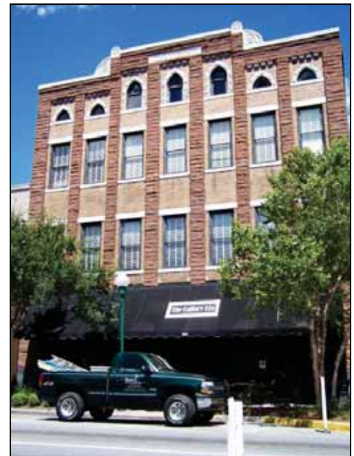
Converse Building at 121-123 N. Patterson Street.
