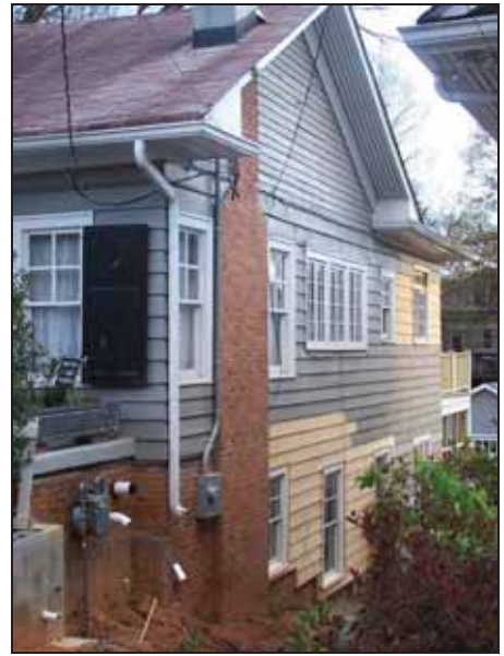
Small sections and individual boards of deteriorated wood siding should be replaced, rather than an entire façade.
