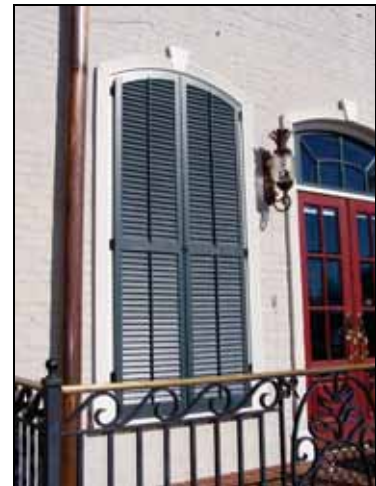
Appropriate shutters cover the entire window.
