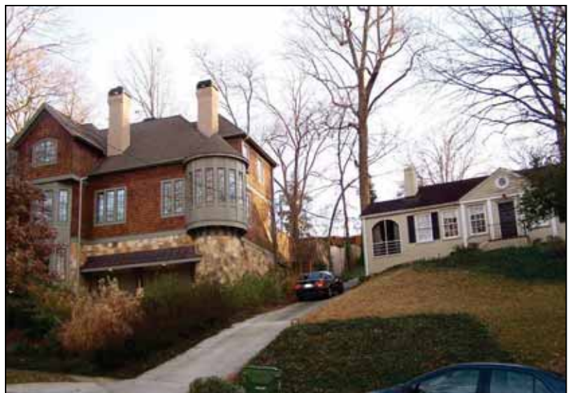
Inappropriate, out-of-scale new construction.
