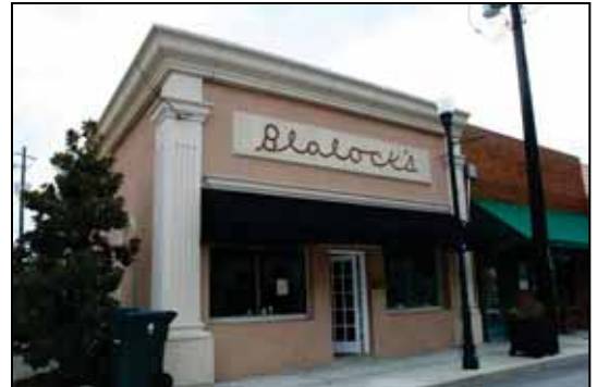
Stucco should not be applied over historic brick.
