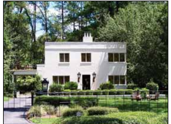
International style house designed by Lloyd Greer.
