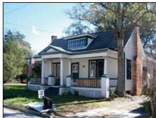
Central Hallway Cottage at 113 North Avenue.
