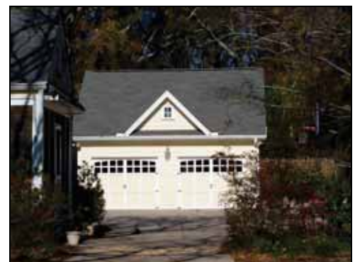
Appropriate design for a new garage.
