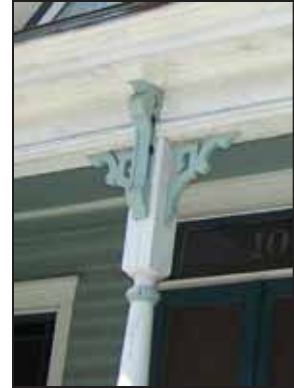
Appropriately maintained porch support with decorative bracket.
