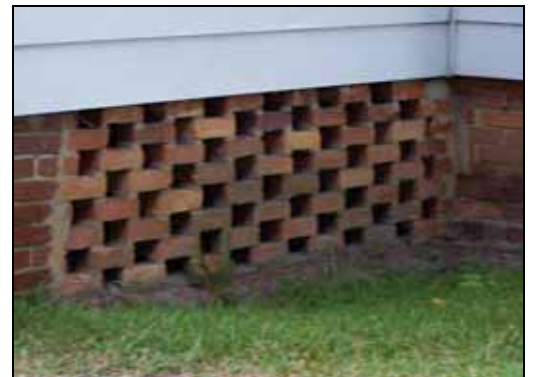
Appropriate maintenance of historic brick latticework infill.
