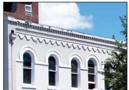
Historic cornices should be maintained and retained.
