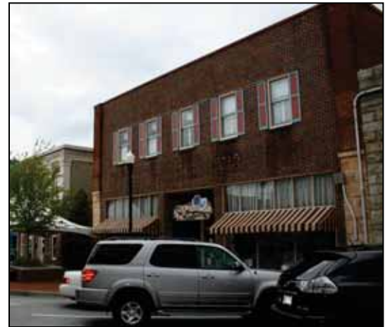
Inappropriate use of shutters.
