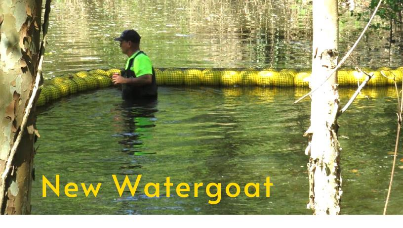
The Stormwater Division of the Engineering Department was happy to receive a much-needed upgrade to the existing Watergoat serving Sugar Creek. This upgraded installation is equipped with larger marine-grade buoys and a double-row configuration to catch floatable debris and litter more effectively. It's important that the community works together to keep the rivers and streams clean.
