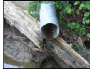
Corrugated Metal Pipe (CMP)
