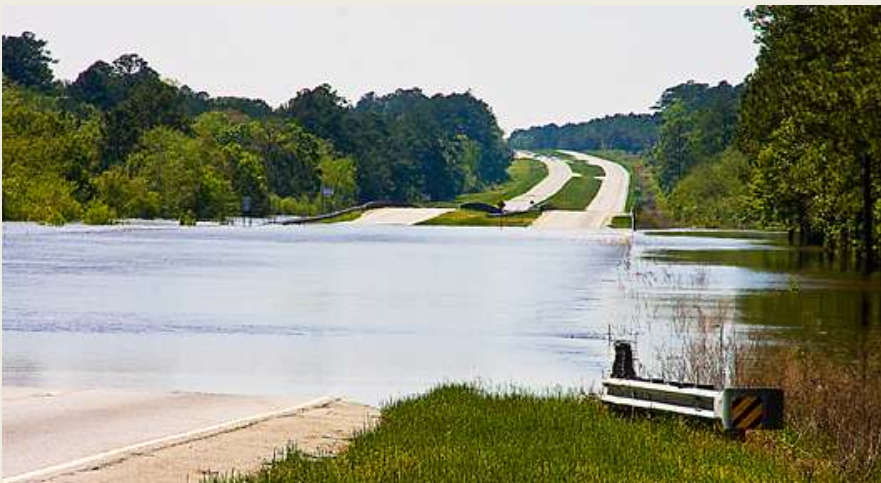
US Highway 84 / Lowndes County Courtesy of Valdosta Daily Times
