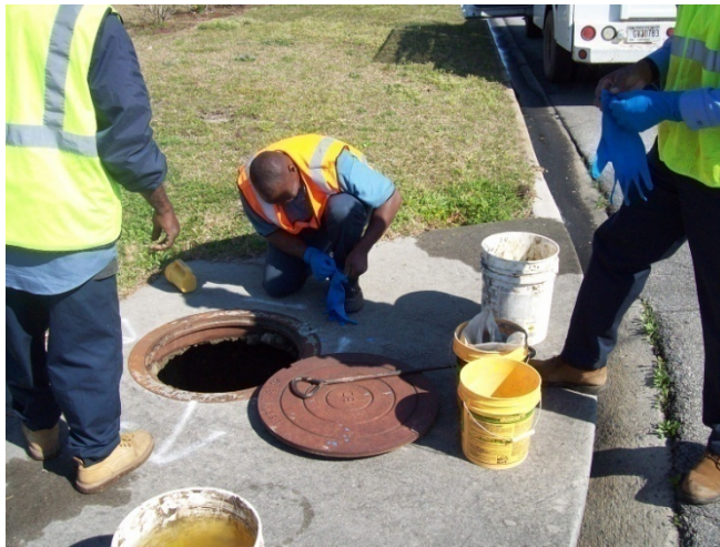
Figure 2: Removing a catch basin manhole lid
