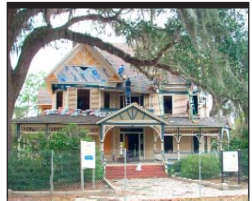
The Roberts House is shown in this January 2012 photo with a new roof and framing.
