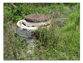
Some Mud Creek Outfall Manholes are in Poor Condition
