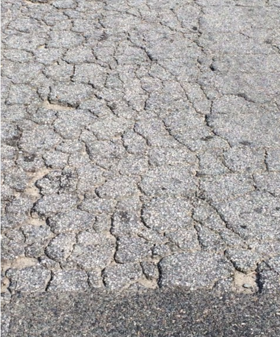
Alligator Cracking
