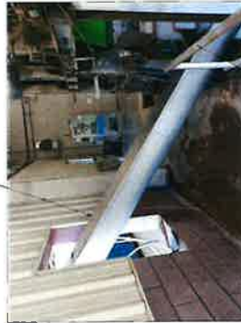
REMOVE AND RELOCATE EXISTING BOOSTER PUMP TO THE NEW BELT FILTER PRESS
